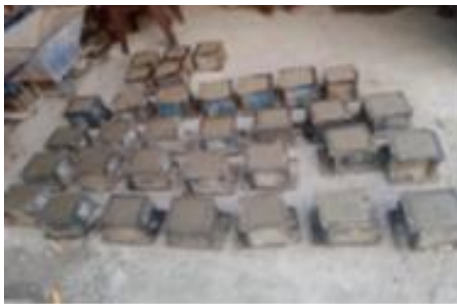
Figure 8: Casting of Cube Specimens
